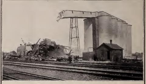
Cut shows H. W. Rogers & Bro.'s Elevator at Harvey, Ill. Operating house burned Sept. 30, 1905. Tile tanks, built by us, with contents were uninjured. This shows the advantages of hollow tile bin construction.
